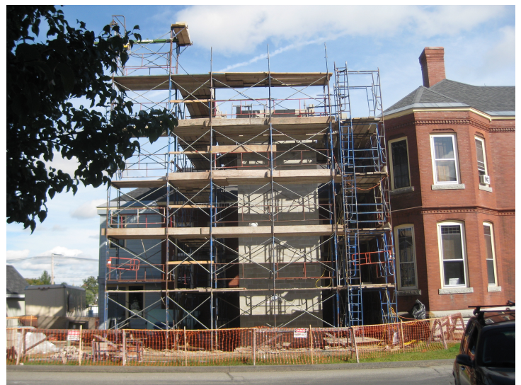
The Elevator Tower!
