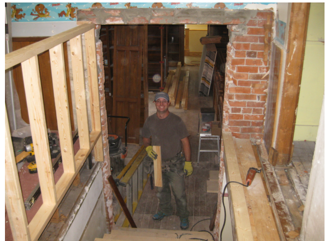
New stairway from second floor down to Mezzanine
