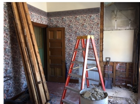
Upstairs bathroom improvements underway!
