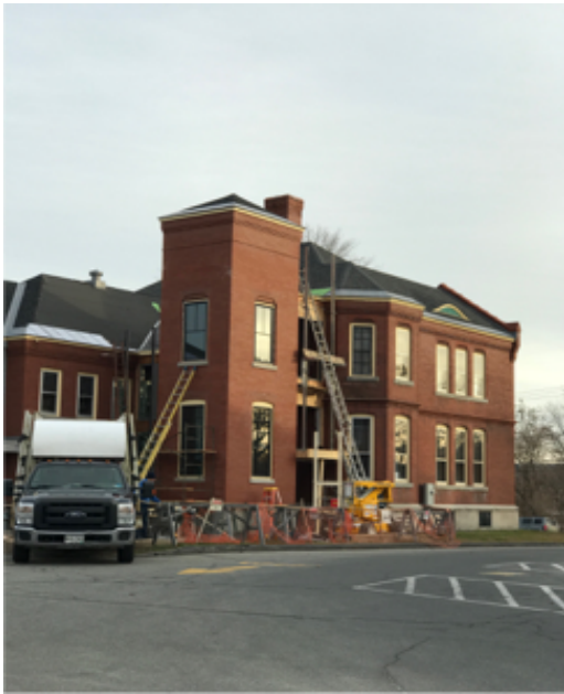
The "almost finished" elevator tower!
