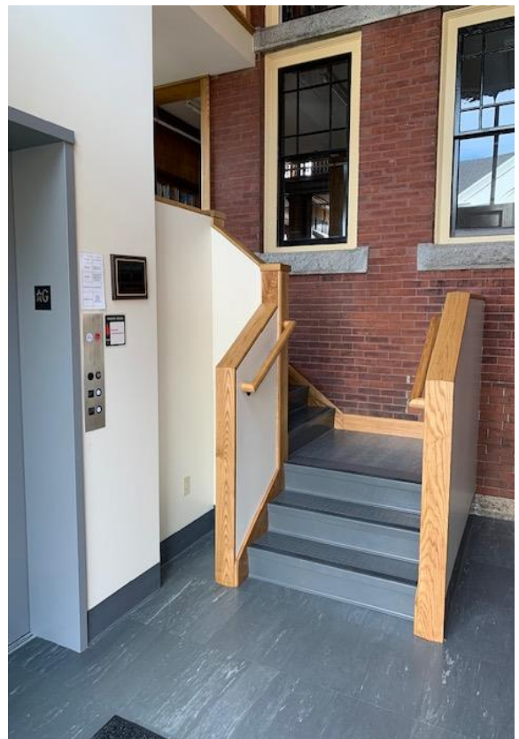
Our beautiful new elevator entrance stairs.
