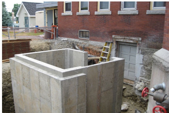
Elevator Foundation!
