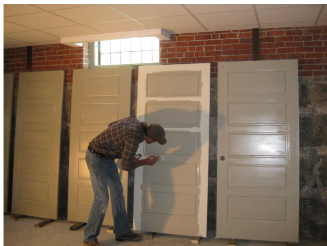
Doors and trim in the basement are painted "Intelligent Gray"
